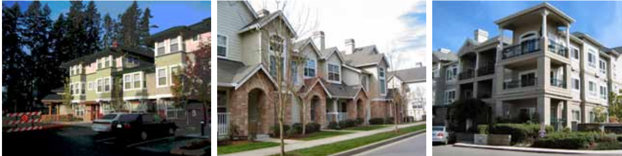
The site plan assumes a combination of walkup apartments (left), town homes (center), and low-rise apartment buildings.
