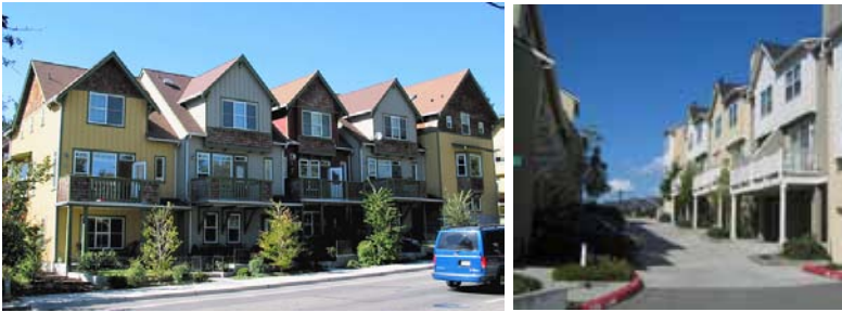
Left image – example of townhouses from street; Right image includes townhouses from private internal court; note planting strips in front of each unit.
