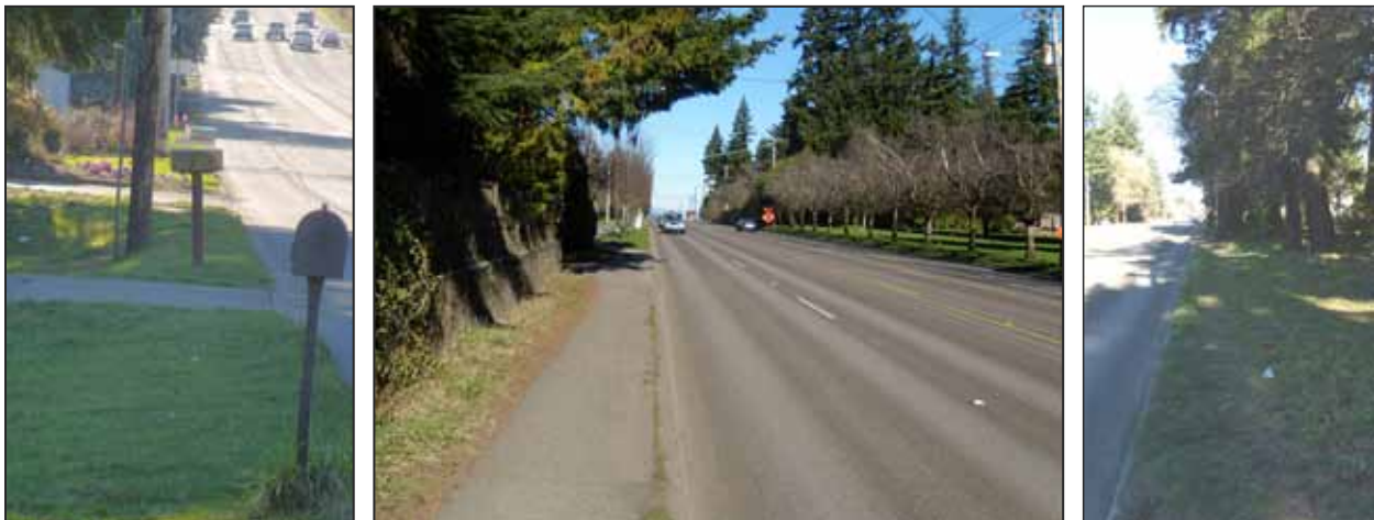
Areas of 112th Avenue with narrow sidewalk or no sidewalk
