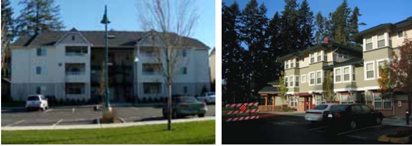
Walk-up apartment examples – Mission Hills building on the left. Image on the right shows a good example with landscaping.
