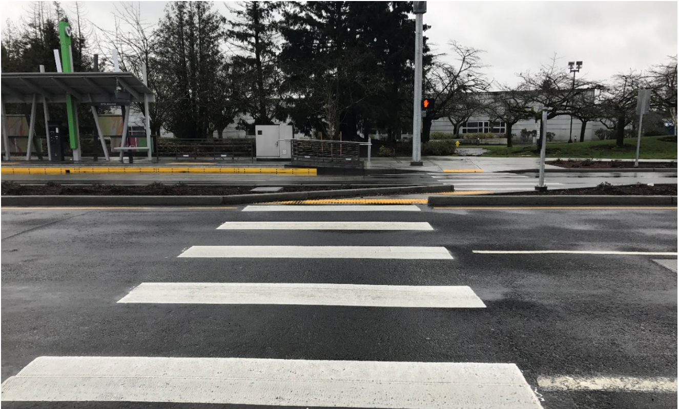
Figure 23. Existing raised median and offset crossing at the 5900 Block Hybrid Beacon
