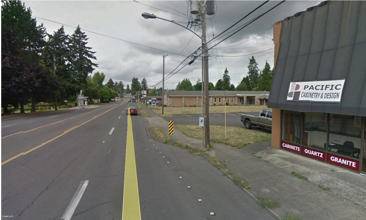
Figure 16: Example of pedestrian through way being obstructed. (Image from Google Streetview)
