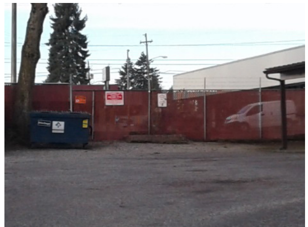
Fence between residential parking lot and commercial parking lot on Fourth Plain Boulevard (Facing North)
