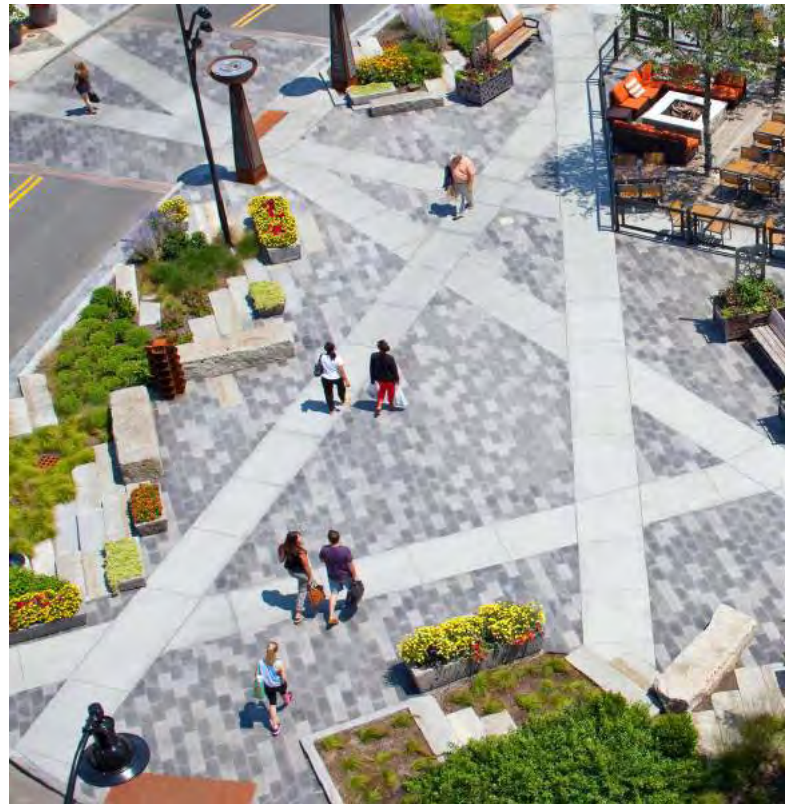
BRICK PAVING + CONCRETE BANDS (LOWER PLAZA)
