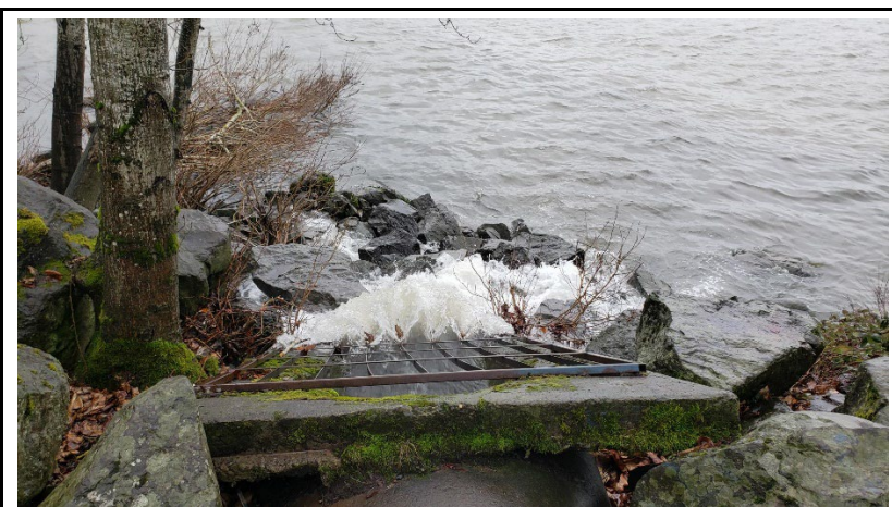
Outfall monitoring station CSP1 – 12/27/2022
