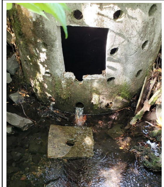
Monitoring stations CSE1 and CSE2 – 1/9/2024 (above). Monitoring station CSE3 – 9/7/2023 (below).
