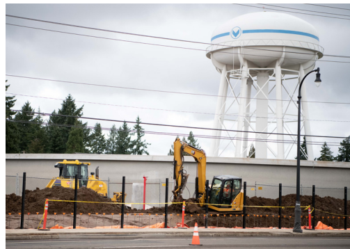
Improvements at Water Station 5 increased capacity and reliability
