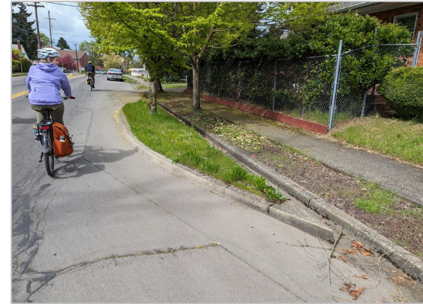
Figure 7. Existing Bulb Out on 33rd Street
