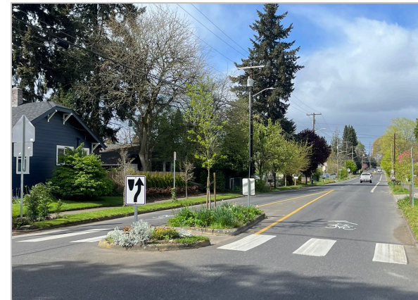
Figure 5. Existing Pedestrian Median Islands on 33rd Street
