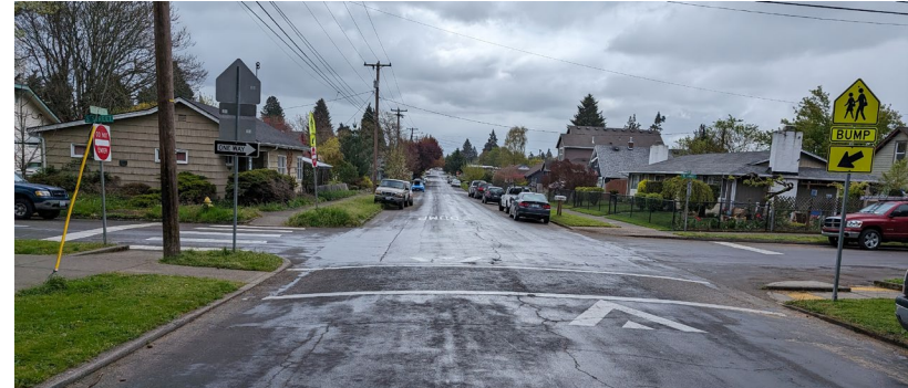
Figure 2: A raised crosswalk at S Street helps slow traffic for students crossing 29th Street.
