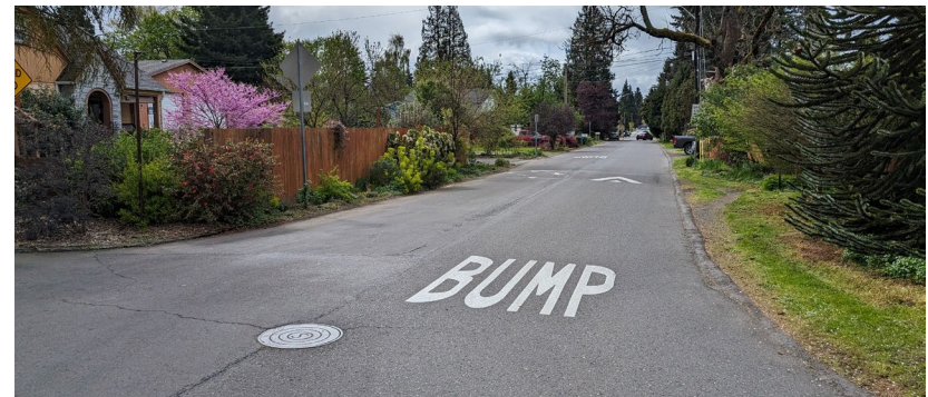
Figure 3: Speed bumps provide traffic calming on the eastern end of the study corridor.
