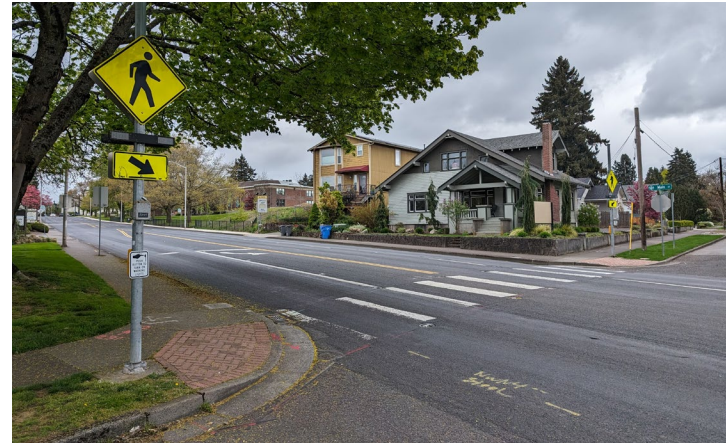
Figure 14: At 29 th Street and Main Street, a continental crosswalk and rectangular rapid flashing beacon (RRFB) are located on the north intersection leg. Coordination with the Upper Main Street project will help identify intersection approach options along 29 th Street.
