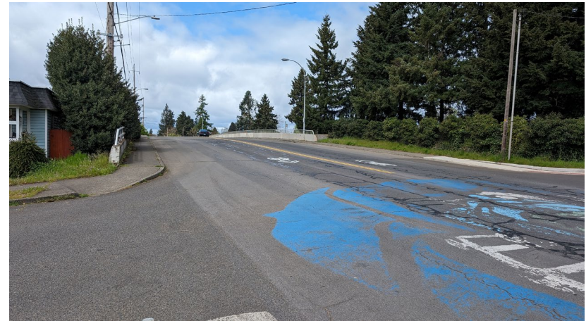
Figure 5: The I-5 Overpass is wide, with sharrows and attached sidewalks.
